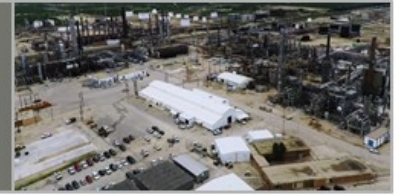
Big Spring Alon Refinery
